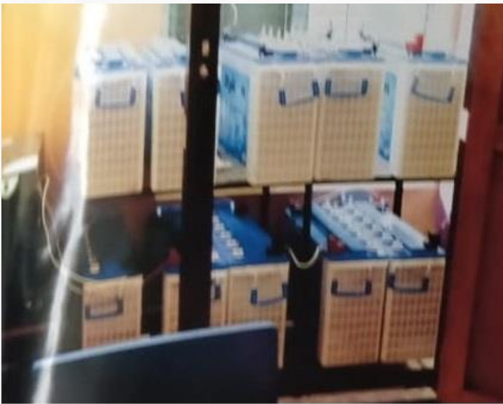
5 kV UPS 120 AH TEN BATTERIES
