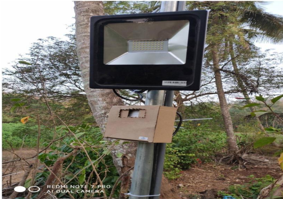
Fig.6 50 watt led light and siren
