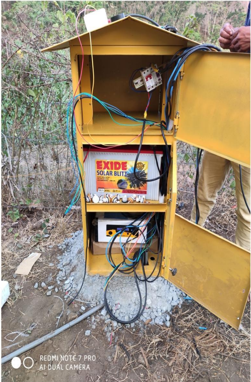
Fig 4. Kiosk box with battery, inverter smart server
